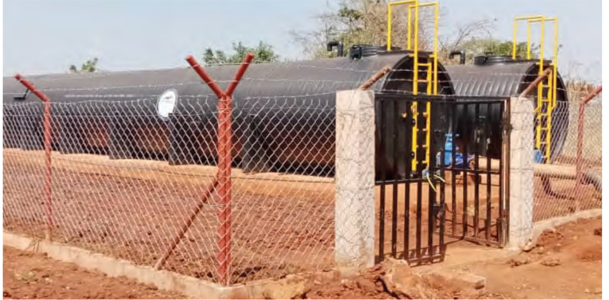
The 300,000 litre Weholite Tank fully installed and safely secured.
