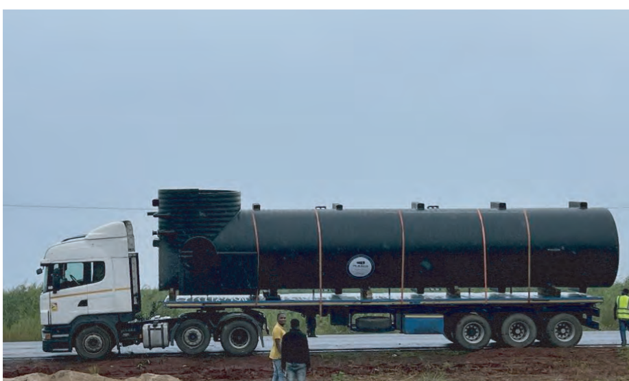
Delivery of the first, factory fabricated tank section.
