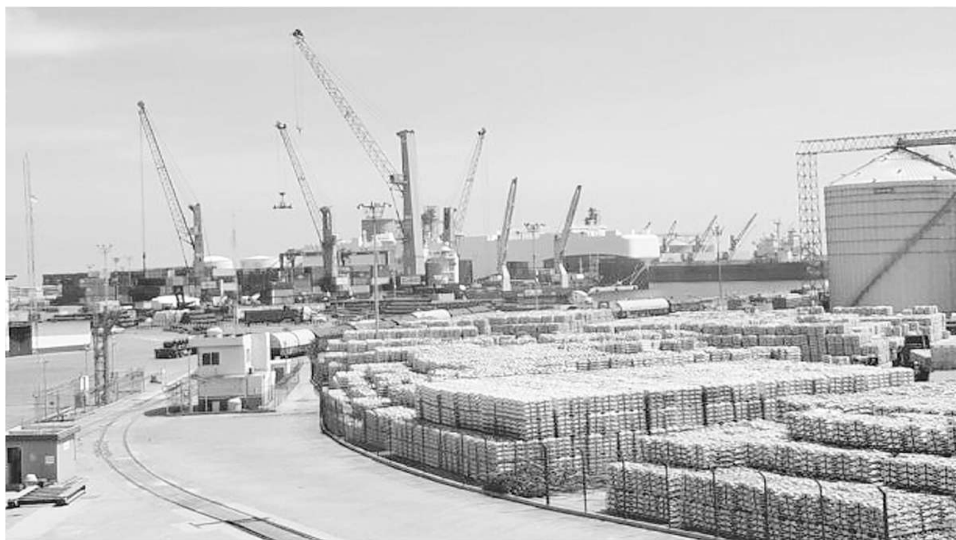
Manoeuvres in the port of Veracruz, in the south-eastern state of the same name and Mexico's third largest. Large port facilities in the country have taken some measures to reduce pollution from their activities, but they are not enough to have clean and sustainable ports.
