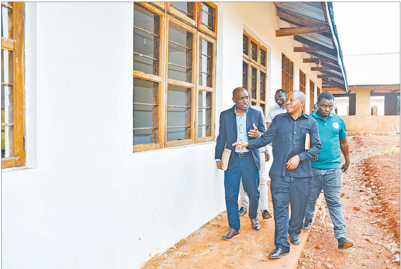
Masozi Nyirenda (L), Tanzania Education Authority's Director of Fundraising and Project Management, pictured yesterday making an inspection tour of progress in the implementation of a science laboratory project at Kasulu District's Nyakitonto Secondary School. Photo: Guardian Correspondent
