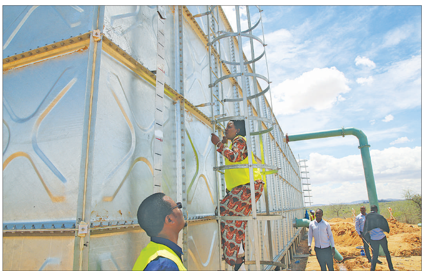
Dodoma regional commissioner Rosemary Senyamule goes up the ladder to inspect a newly built three-million-litre water tank in Dodoma Urban District's Nzuguni administrative ward yesterday. Left is Dodoma Urban Water Supply and Sanitation Authority engineer Aron Joseph. Photo: Correspondent Ibrahim Joseph
