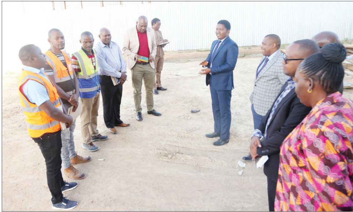
Minister of State in the Vice President's Office (Union and Environment) Dr Selemari Jafo (C) talks with contractors and the ministry's officials after visiting the construction site of Vice President's Office in Dodoma yesterday. Photo: VPO
