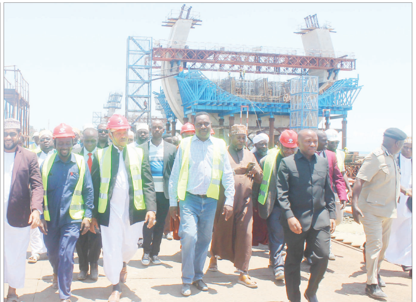
Dar es Salaam regional commissioner Abubakari Kunenge (C) leads religious leaders on Monday during an inspection tour of Tanzanite Bridge, which is under construction. It will link the city's Upanga-Seaview and Oysterbay areas. Photo: Correspondent Jumaine Juma
