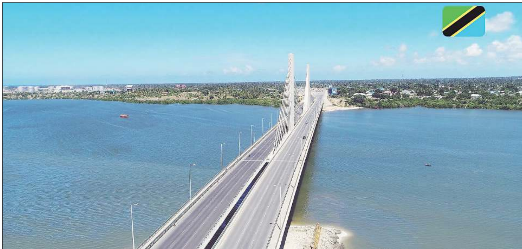
Kigamboni's Nyerere Bridge has made the new municipality a popular place for developers hence fuelling land conflicts. File photo.
