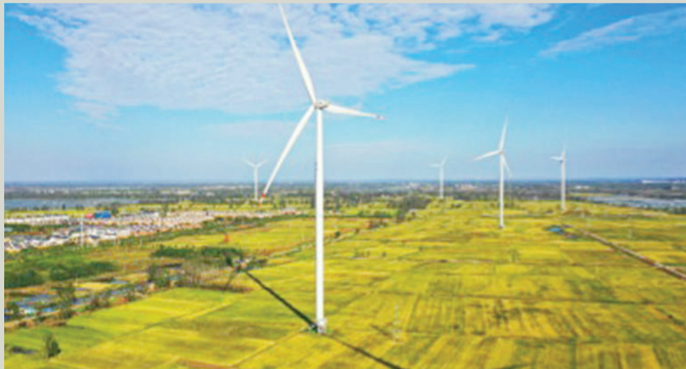
Photo shows wind turbines at a wind farm in Weiji township, Suining county, Xuzhou city, east China's Jiangsu province, Oct. 11, 2021. File photo
