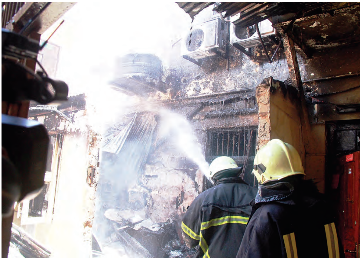
Fire and Rescue Force officers extinguish the blaze at a house located on the storey building at the junction of India Street and Morogoro Road in Dar es Salaam yesterday. There were no casualties. Photo: Correspondent Jumanne Juma
