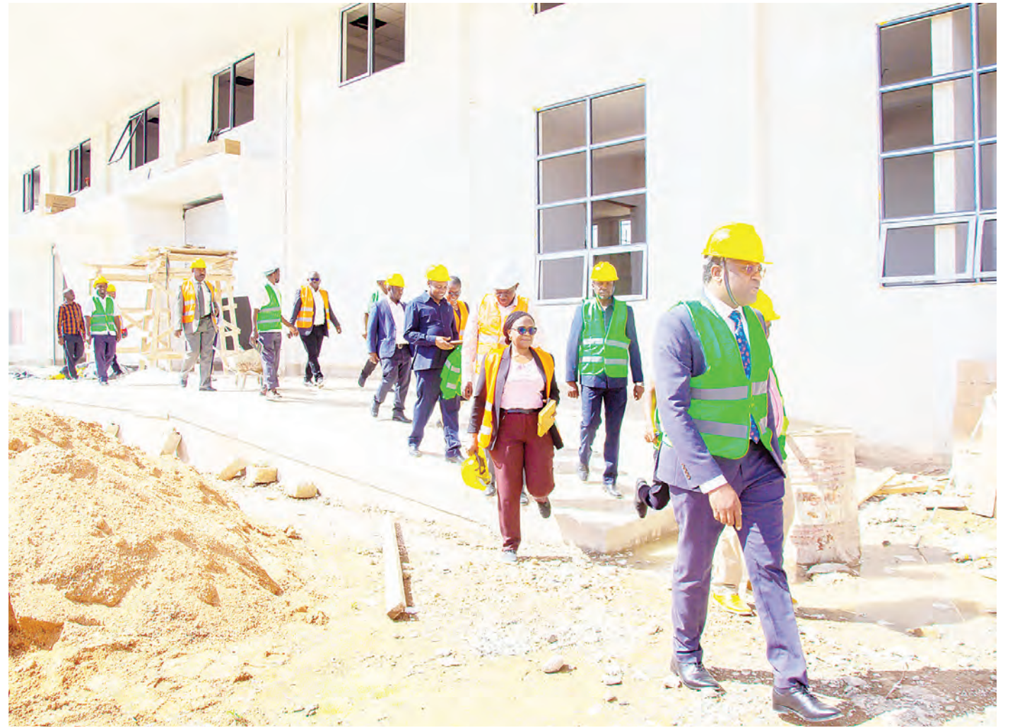
Permanent secretary in the Prime Minister's Office (Policy Parliament and Coordination) Dr Jim Yonazi (R) inspects the progress of the construction of government chief printer office building at Kisasa area in Dodoma on Thursday. Photo: Correspondent Peter Mkwavila
