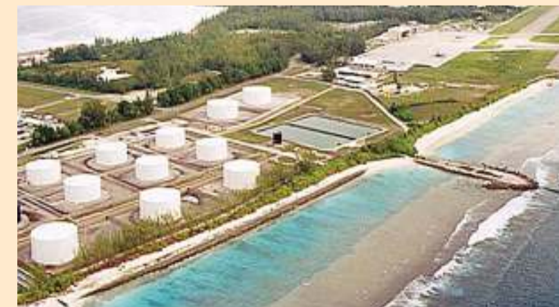
Fuel tanks on Diego Garcia, the largest island in the Chagos archipelago and the site of a US military base.
