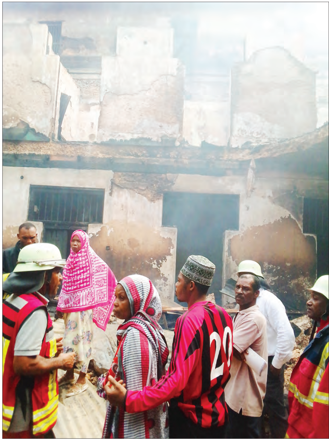
Residents of Kiponda Street in Zanzibar look on helplessly at the debris of a building gutted by fire at midnight yesterday, leaving scores of families homeless. Photo: Correspondent Martin Kabemba
