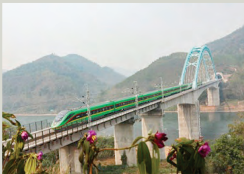
Train D887 runs on a bridge along the China-Laos Railway in Jinghong, southwest China's Yunnan province, April 13. (Photo by Li Yunsheng/People's Daily Online)
