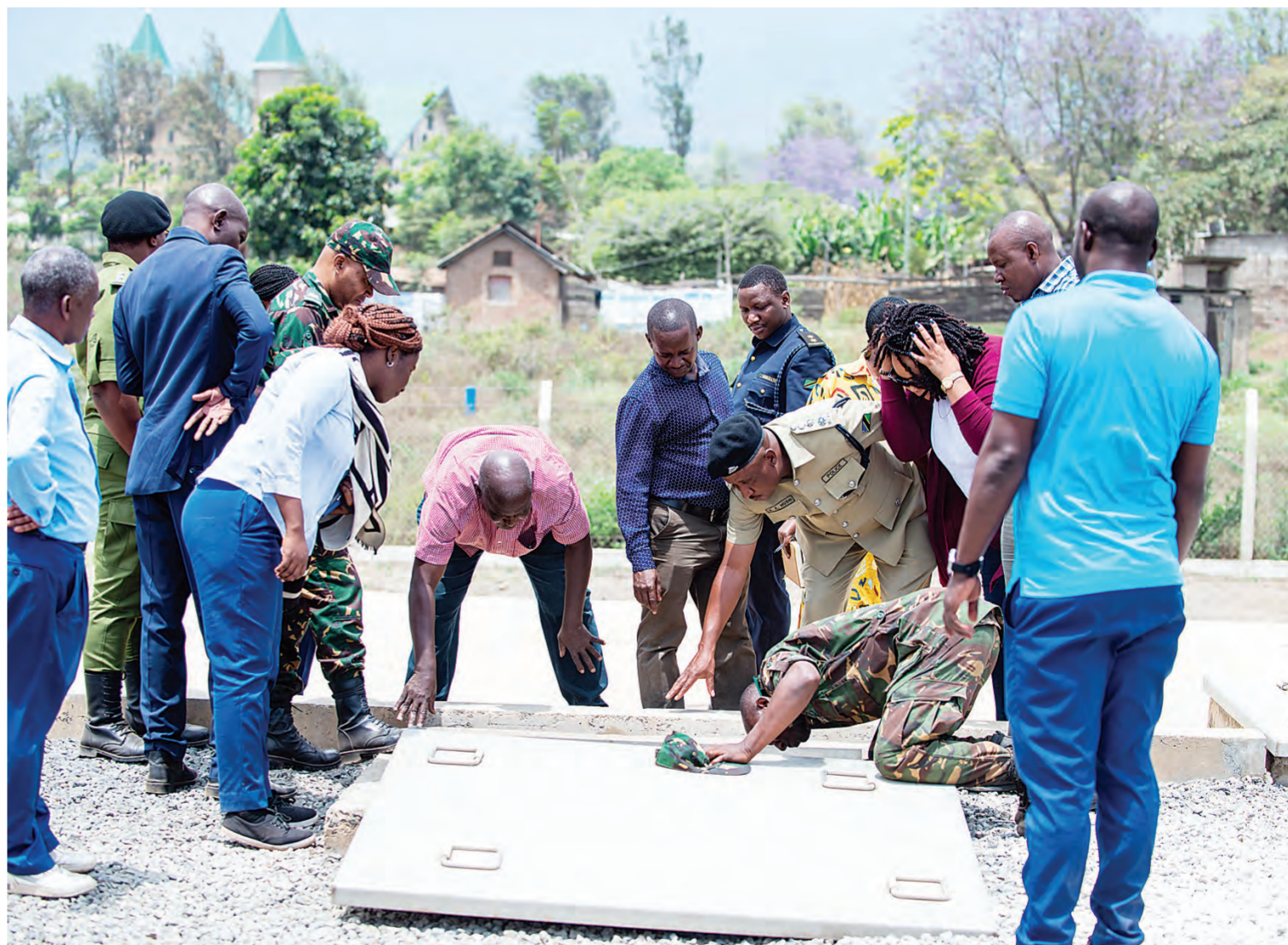
Members of the Arusha District defence and security committee and Arusha Urban Water and Sanitation Authority staff check an underground tank at Ngarantoni yesterday during an inspection tour of water sources. Photo: Correspondent Getrude Mpenzya
