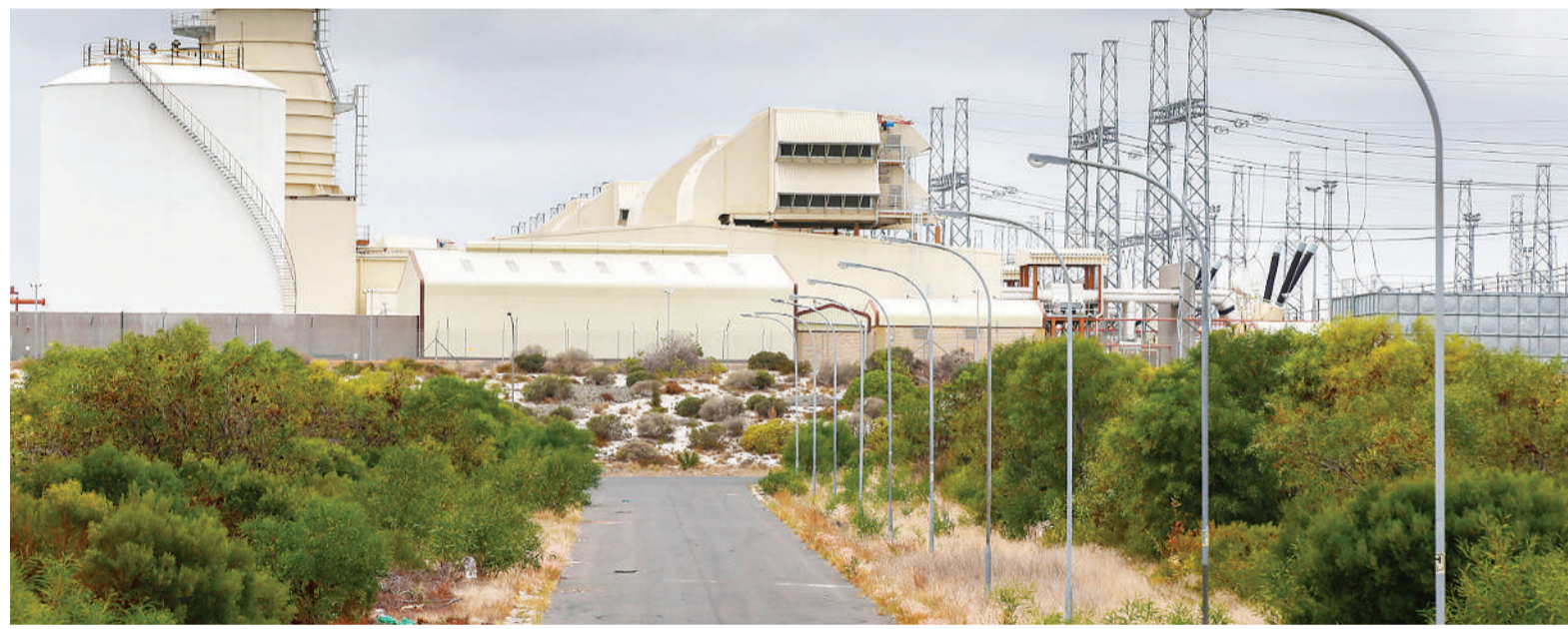
Ankerlig power station in Atlantis outside Cape Town. EPA/NIC BOTHMA
