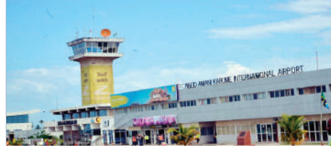
ABEID AMANI KARUME AIRPORT CONSTRUCTION PAGE 6
