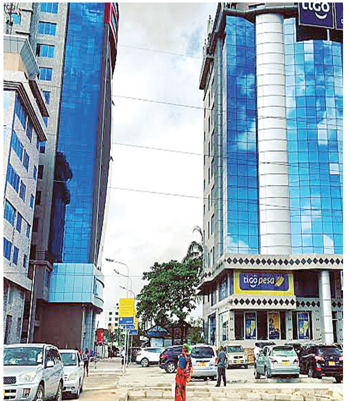
A complex where Tigo is headquartered in Dar es Salaam. File photo.
