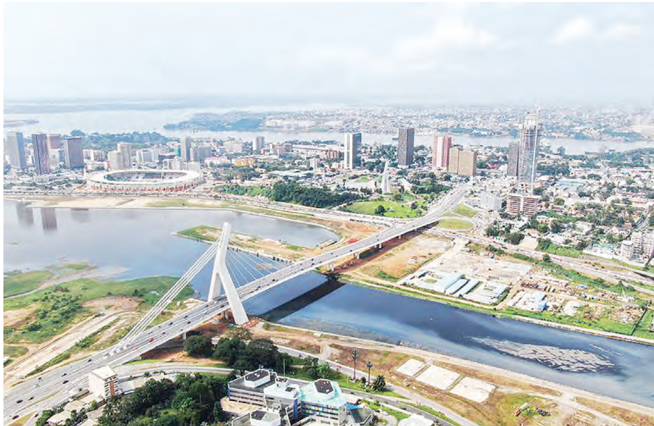
This aerial photo taken on Jan. 9, 2024 shows a view of Cocody Bridge in Abidjan, Cote d'Ivoire. Xinhua
