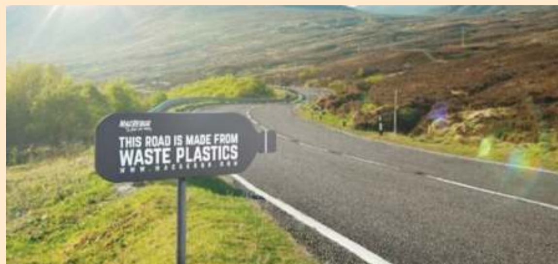
Construction of a plastic road in Kouga Municipality in the Eastern Cape.
