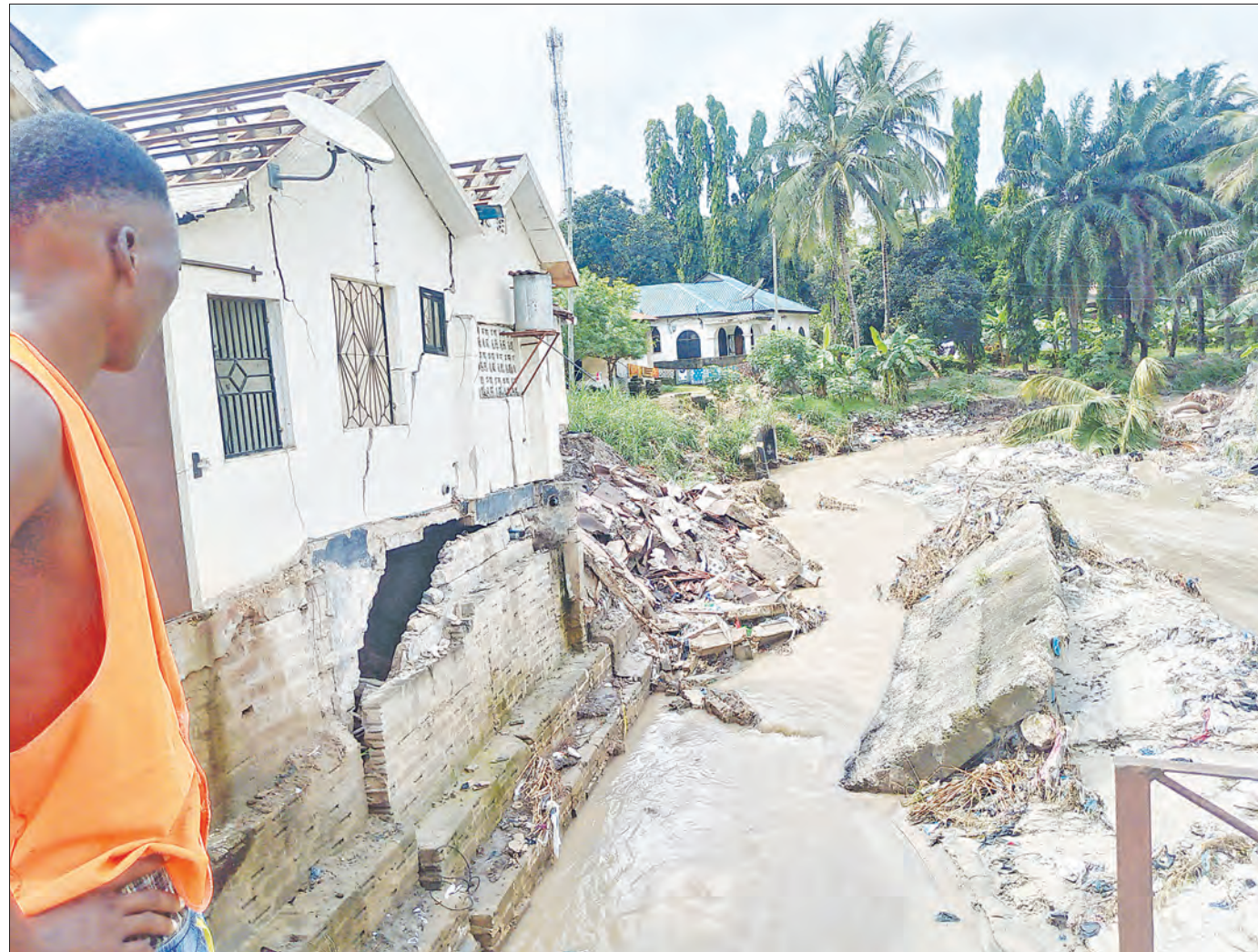
RAIN-INDUCED DANGER: A resident of Msigani in Dar es Salaam's Mbezi Luis suburb looks on helplessly yesterday at a house in clear danger of crumbling, with floodwaters courtesy of the ongoing heavy rains having burst the banks of the small river it borders. Photo: Correspondent Sabato Kasika
