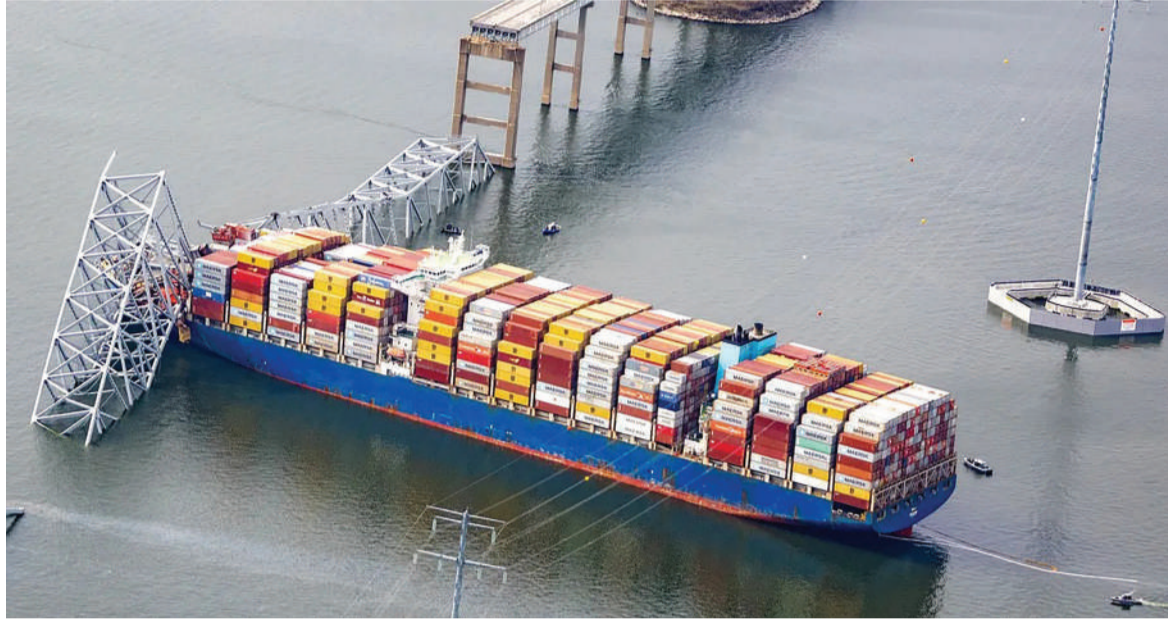
A cargo ship 'Dali,' crashed into the Francis Scott key bridge in US on March 26, 2024. Photo: Tasos Katopodis / Stringer/Getty Images
