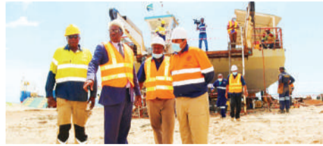
MV MAFANIKIO REPAIR NEARS COMPLETION PAGE 5
