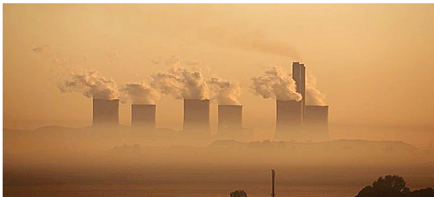
Steam rises at sunrise from the Lethabo Power Station, a coal-fired power station owned by state power utility Eskom near Sasolburg, South Africa, 2 March 2016.
