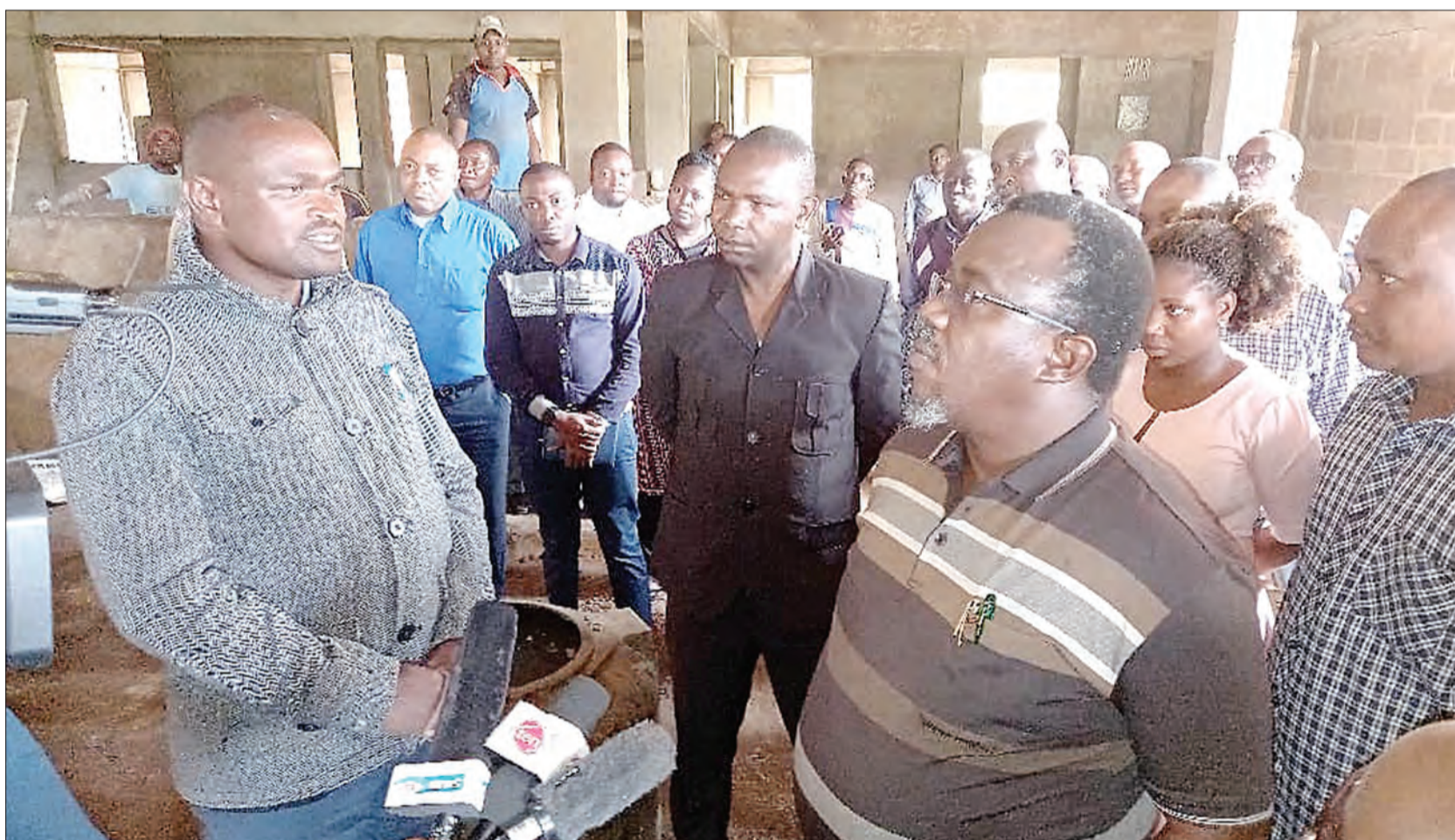
Leonard Mshahara (L), a technician on a team overseeing the construction of a building to house Lushoto District Hospital's mother and child wing, briefs Tanga regional commissioner Adam Malima (in glasses) on Thursday on the ongoing work. The RC was on an inspection tour of Covid-19-related projects in the region. Photo: Correspondent Hamida Kamchalla.
