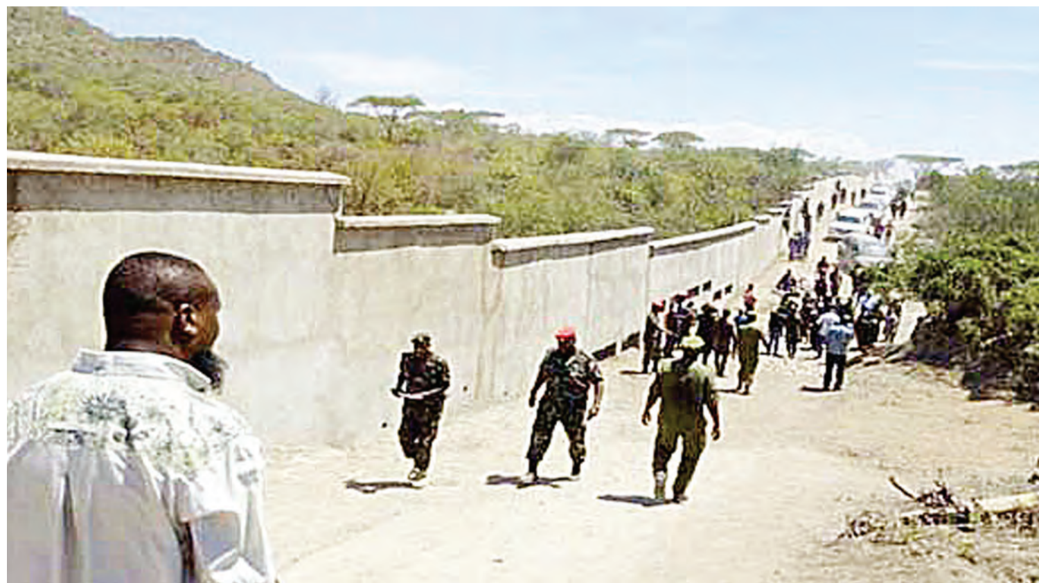
A wall fencing at Mererani tanzanite mines built by the government over two year ago to curb smuggling of the gem.
