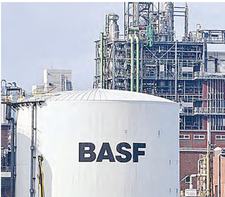
Germany BASF plant
