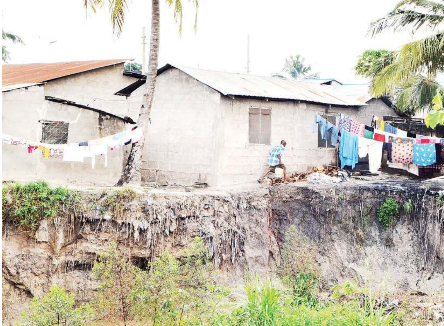
DANGER LURKS: These houses in Dar es Salaam's densely populated Tandale suburb literally stand in harm's way, seriously threatened by soil erosion, as found yesterday. Photo: Correspondent Miraji Msala
