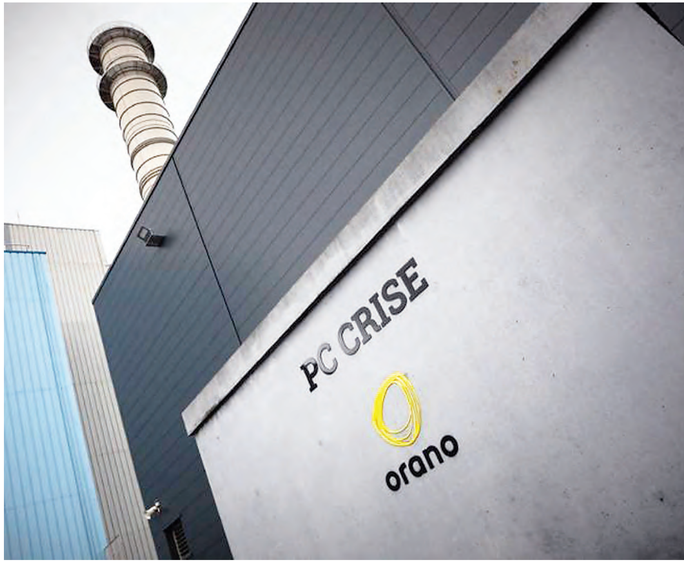
This photo taken on Dec 14, 2022 shows an outdoor view of the crisis unit at the Orano la Hague reprocessing plant, in La Hague, northwestern France, with the Orano logo on a facade. (PHOTO / AFP)
