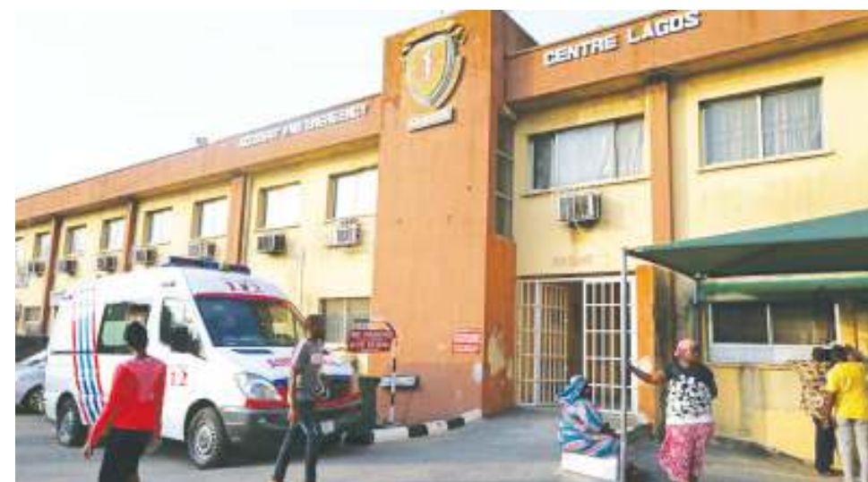
People wait outside a hospital after a building containing a school collapsed in Nigeria's commercial capital Lagos, Nigeria March 13, 2019 [Reuters]
