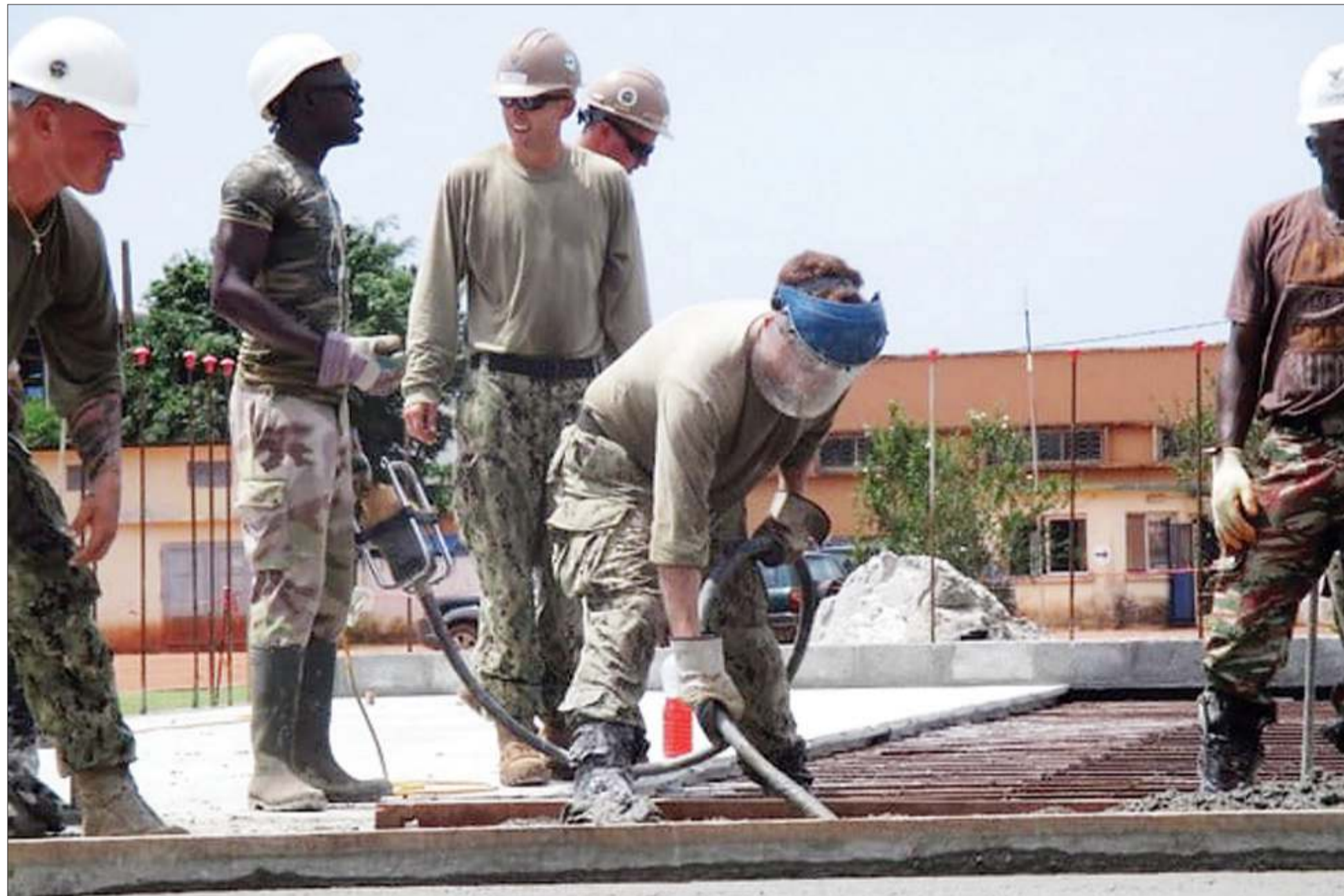
Construction of Gabon's maritime operations centre under way at Port Gentil.
