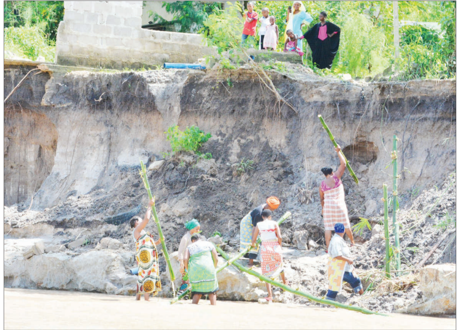
Residents of Dar es Salaam's Goba Matosa suburb plant bamboos on the banks of Mbezi River yesterday in a desperate attempt to prevent soil erosion from further threatening to demolish their houses. Photo: Correspondent Miraji Msala
