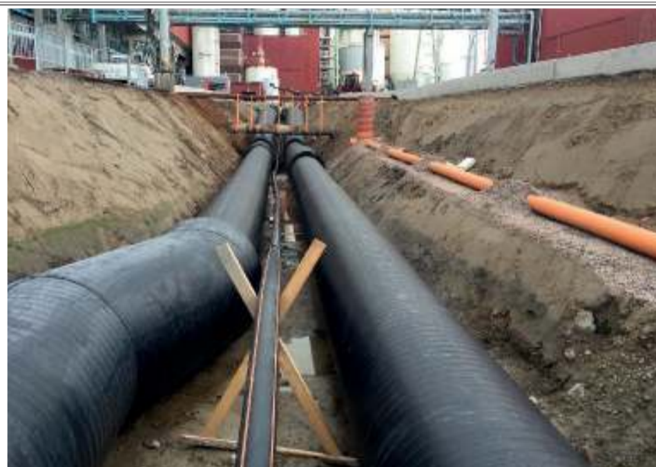
Drainage / Sewerage Systems
