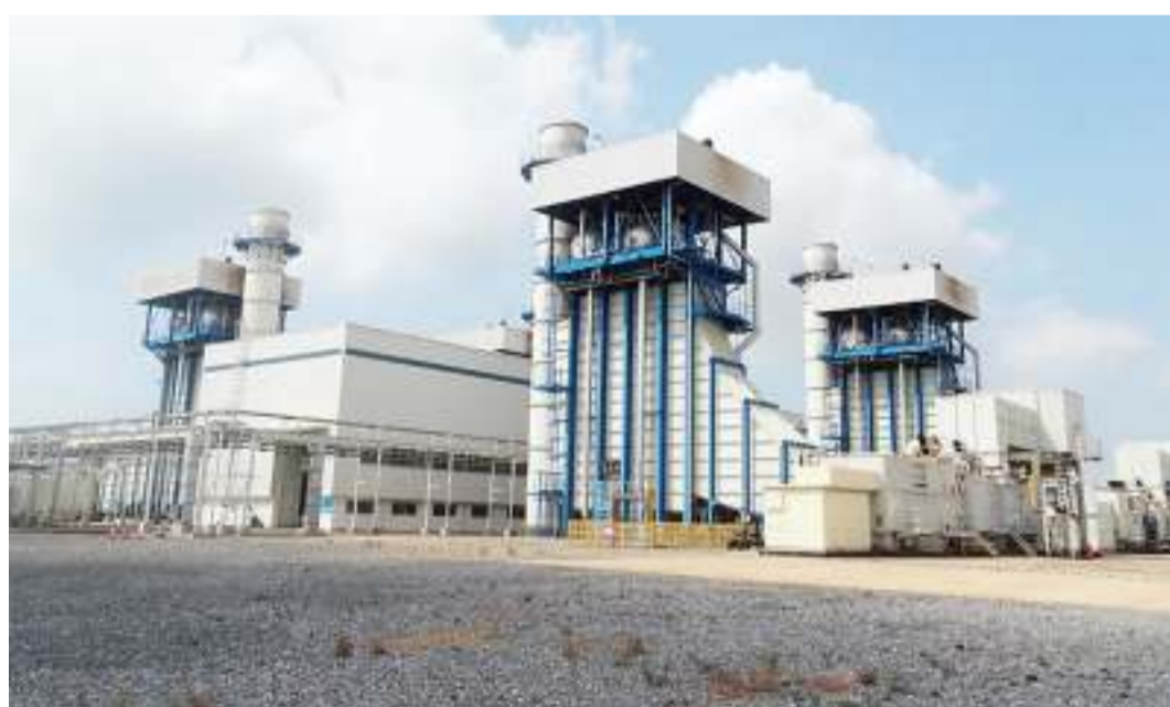
Group Five's Kpone power plant in Ghana
