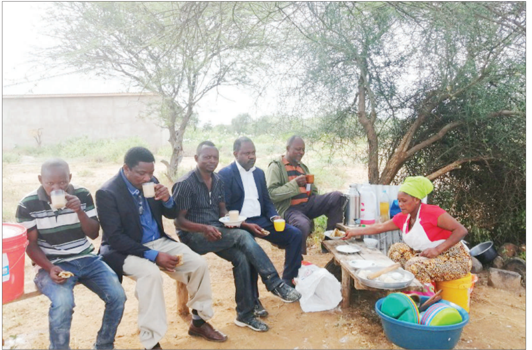
Longido district executive director Juma Mhina (4th-L) has breakfast alongside masons and technicians at the weekend during an inspection tour of the site where a new hospital for the district is being built. Photo: Correspondent Woinde Shizza
