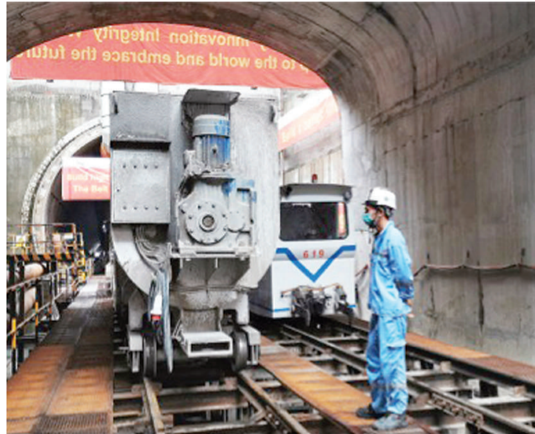
An employee conducts safety inspection for electric carriers at the No. 1 tunnel of the Jakarta-Bandung high-speed railway, Feb. 10. (File photo)
