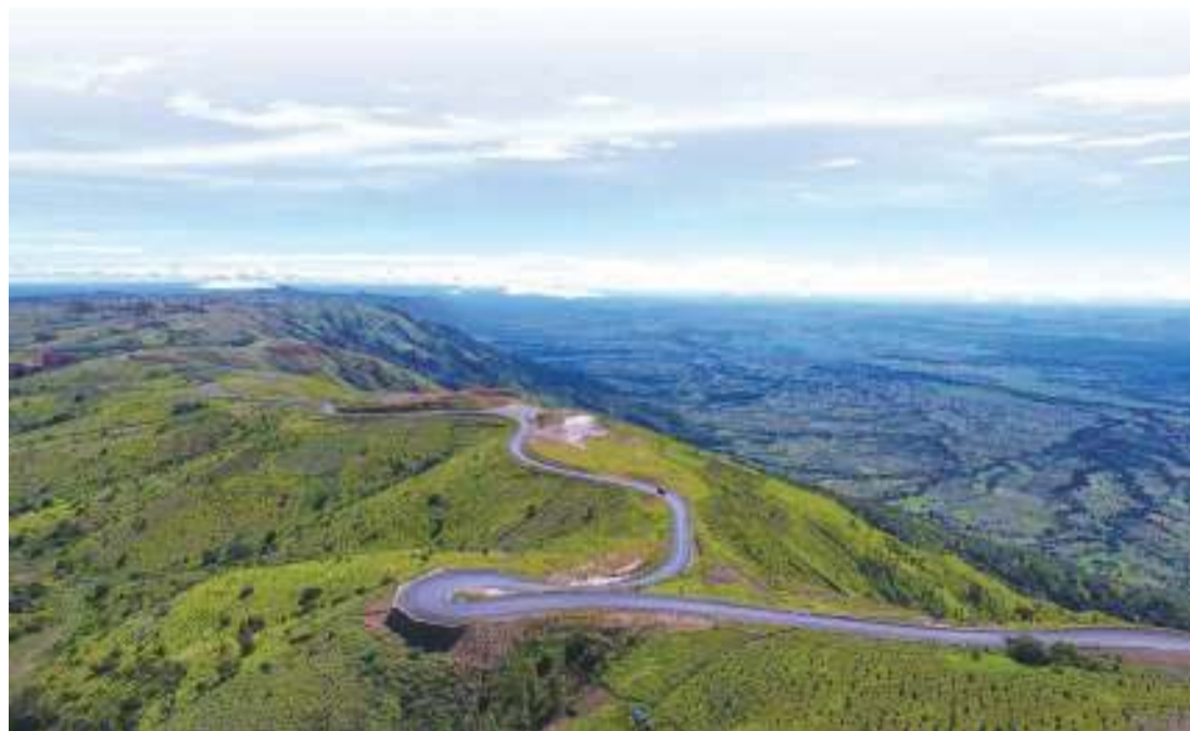
The photo shows the Mbeya-Luwanjiro highway, Tanzania constructed by China Road and Bridge Corporation. Built on an average altitude of 2,000 meters, the highway is the "highest" in the country. Photo by Shi Yue
