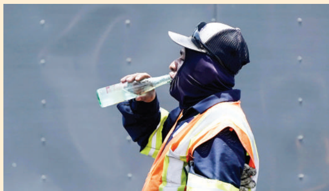
Standing in the mid-afternoon heat, a worker takes a break to drink during a parking lot asphalt resurfacing job in Richardson, Texas, United States, on June 20, 2023. (PHOTO / AP)
