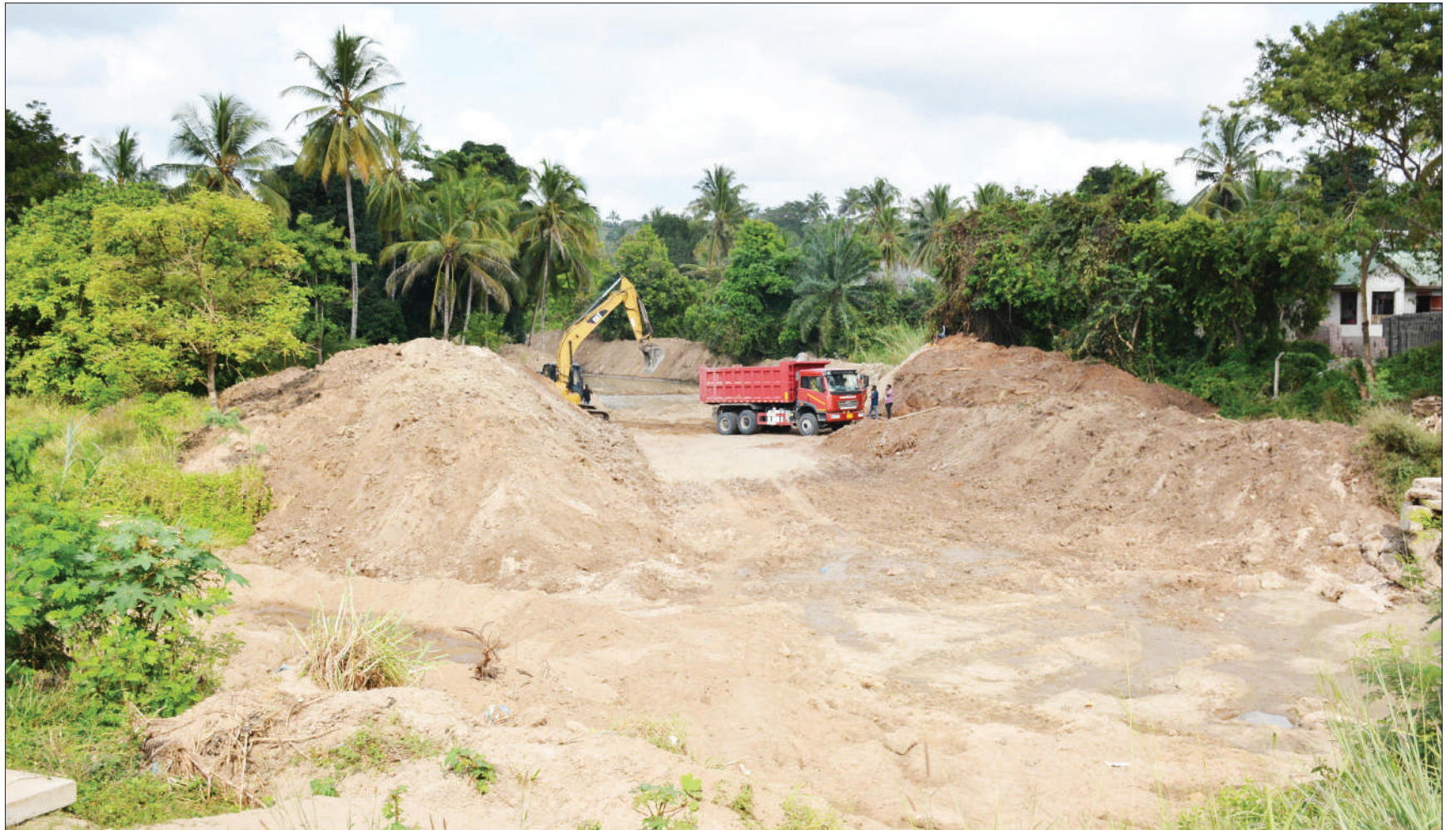
The expansion of Tegeta river is going on at Goba in the outskirts of Dar es Salaam to prevent home flooding. Photo: Correspondent Miraji Msala
