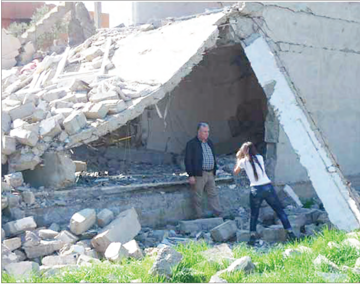
Resident of Hamdaniya district stands before a house destroyed in a Coalition airstrike, February 2017. File photo
