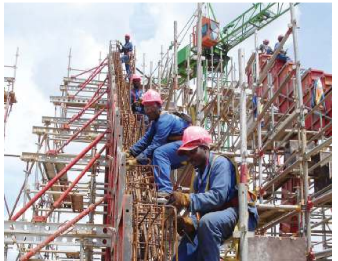
A construction site in Johannesburg.
