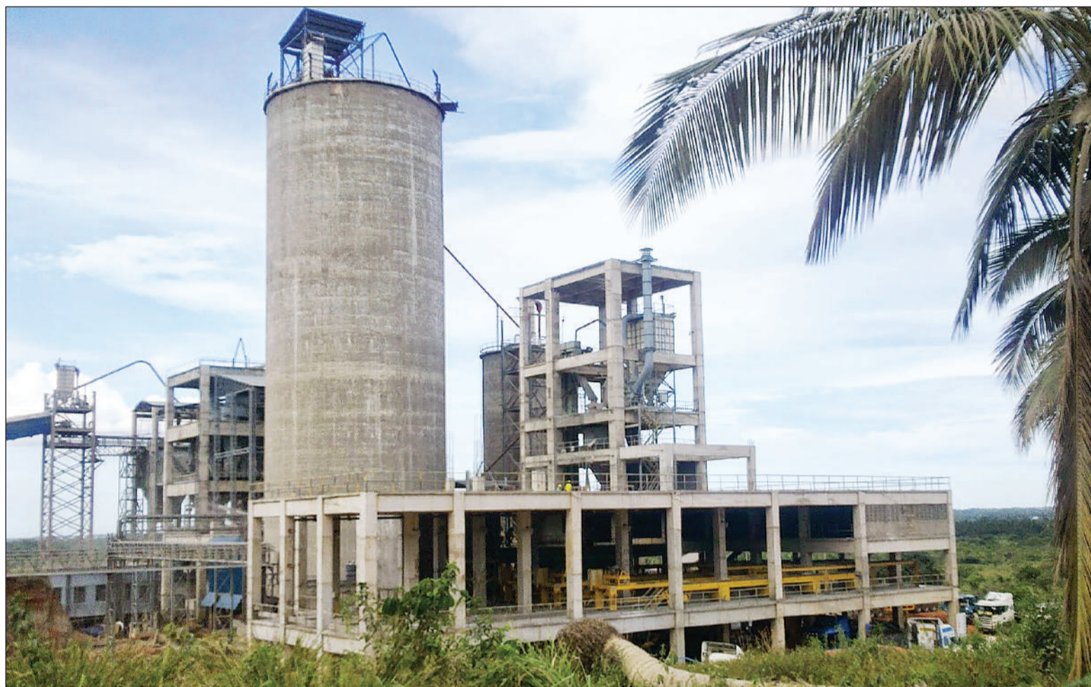
Maweni Limestone Plant in Tanga.
