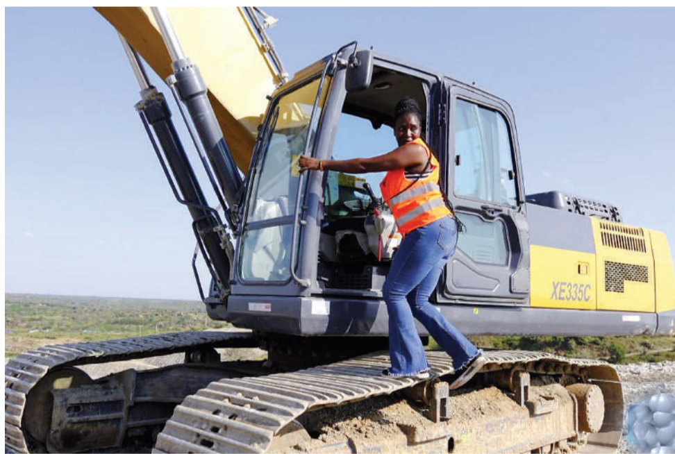
Construction site at Thwake Dam in Makueni, Kenya
