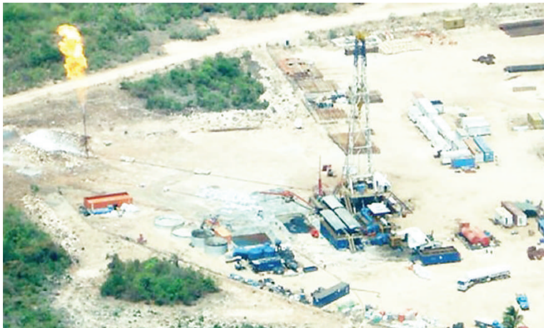
Songas Limited's natural gas plant on Songo Songo Island in Kilwa District.
