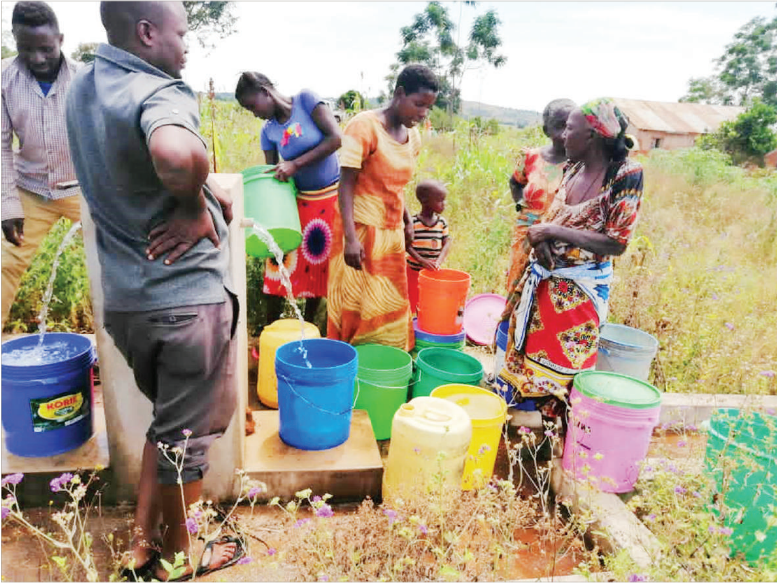
Residents of Busungu and Kwikerege village in Musoma Rural constituency wait for their turns to draw water at a tap installed during yesterday's launch of a Lake Victoria water project. Photo: Guardian Correspondent
