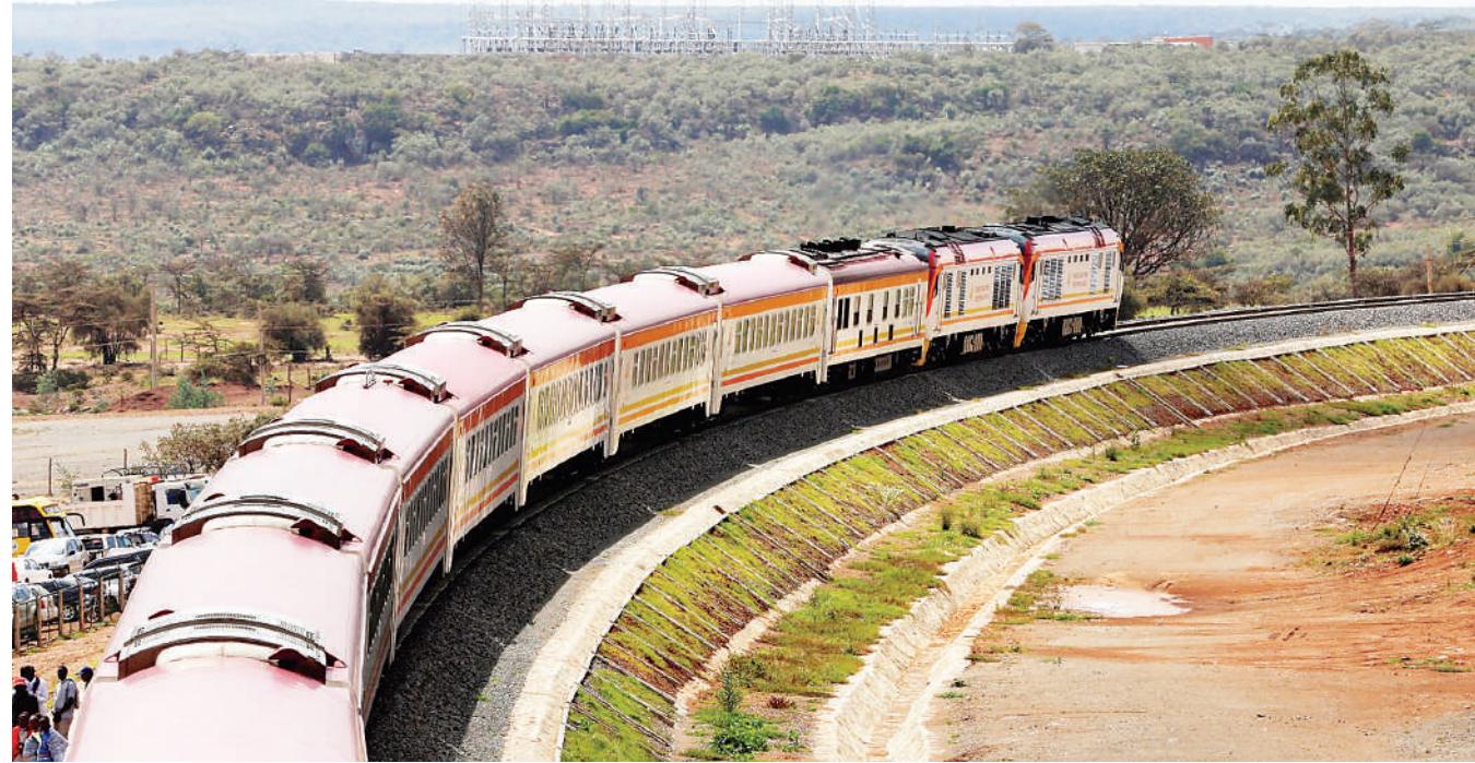
A train on the Standard Gauge Railway (SGR) line in Kimuka, Kenya.
