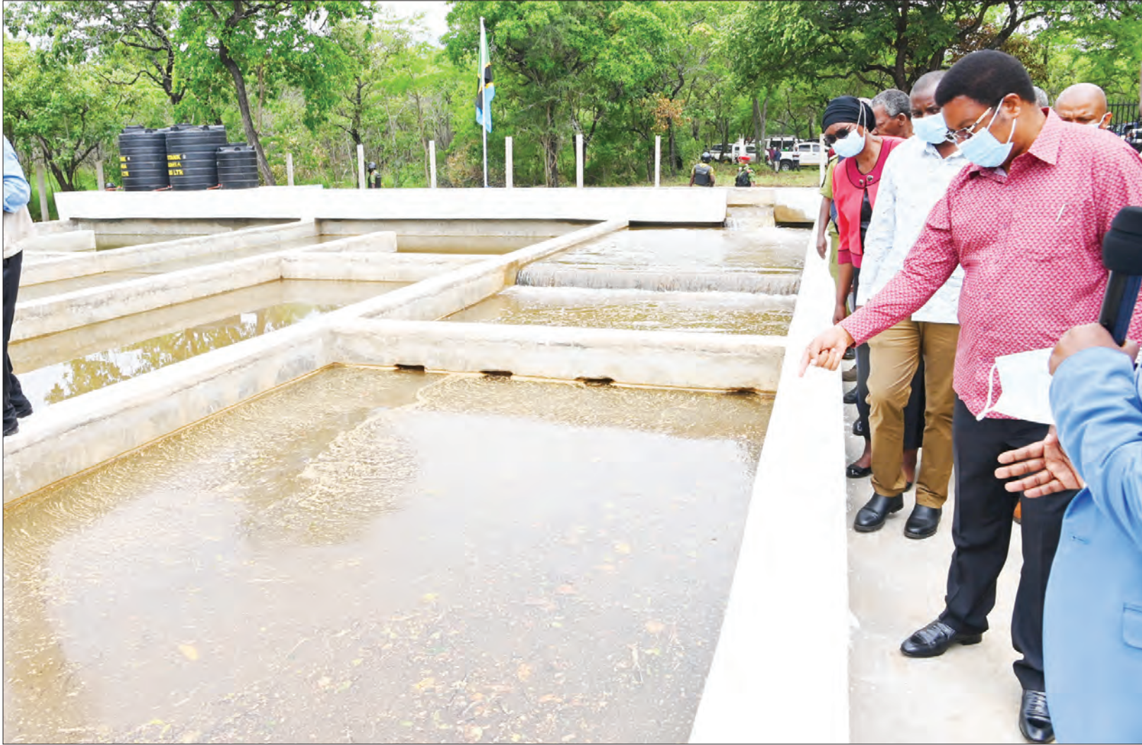
Prime Minister Kassim Majaliwa inspects a water filtering system at the Darakuta-Magugu-Mwada source in Manyara Region's Babati Rural constituency yesterday before laying the foundation stone for the project. Photo: PMO
