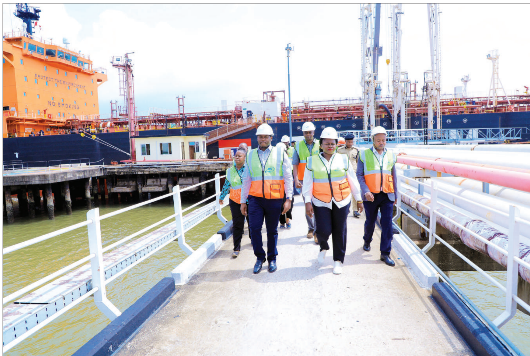
Energy deputy minister Judith Kapinga (C) inspects fuel unloading infrastructure at the Dar es Salaam Port yesterday. Photo: Guardian Correspondent
