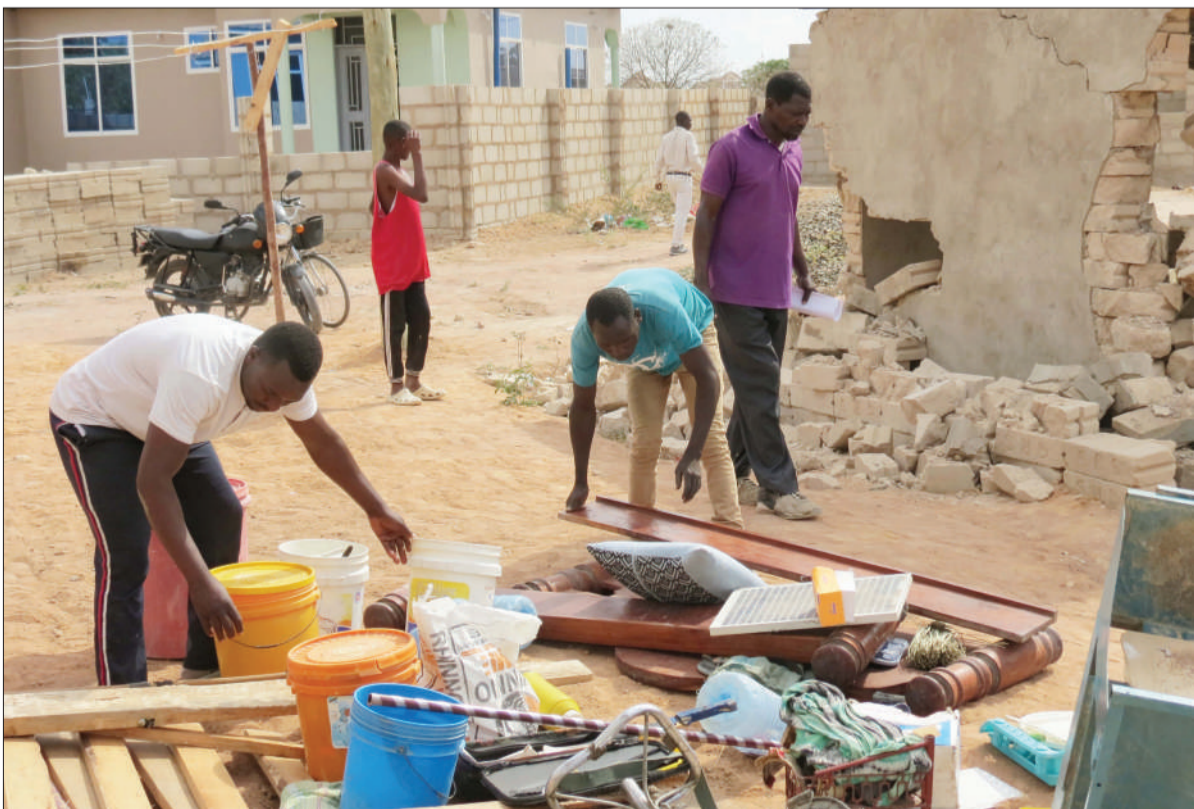
Members of the family of Daud Mpanjilwa of C Centre Street in Nkuhungu ward, Dodoma Urban District, pictured yesterday removing their earthly belonging from what has been their family house but which is said to have been built on what is officially designated as open space. Photo: Correspondent Peter Mkwavila
