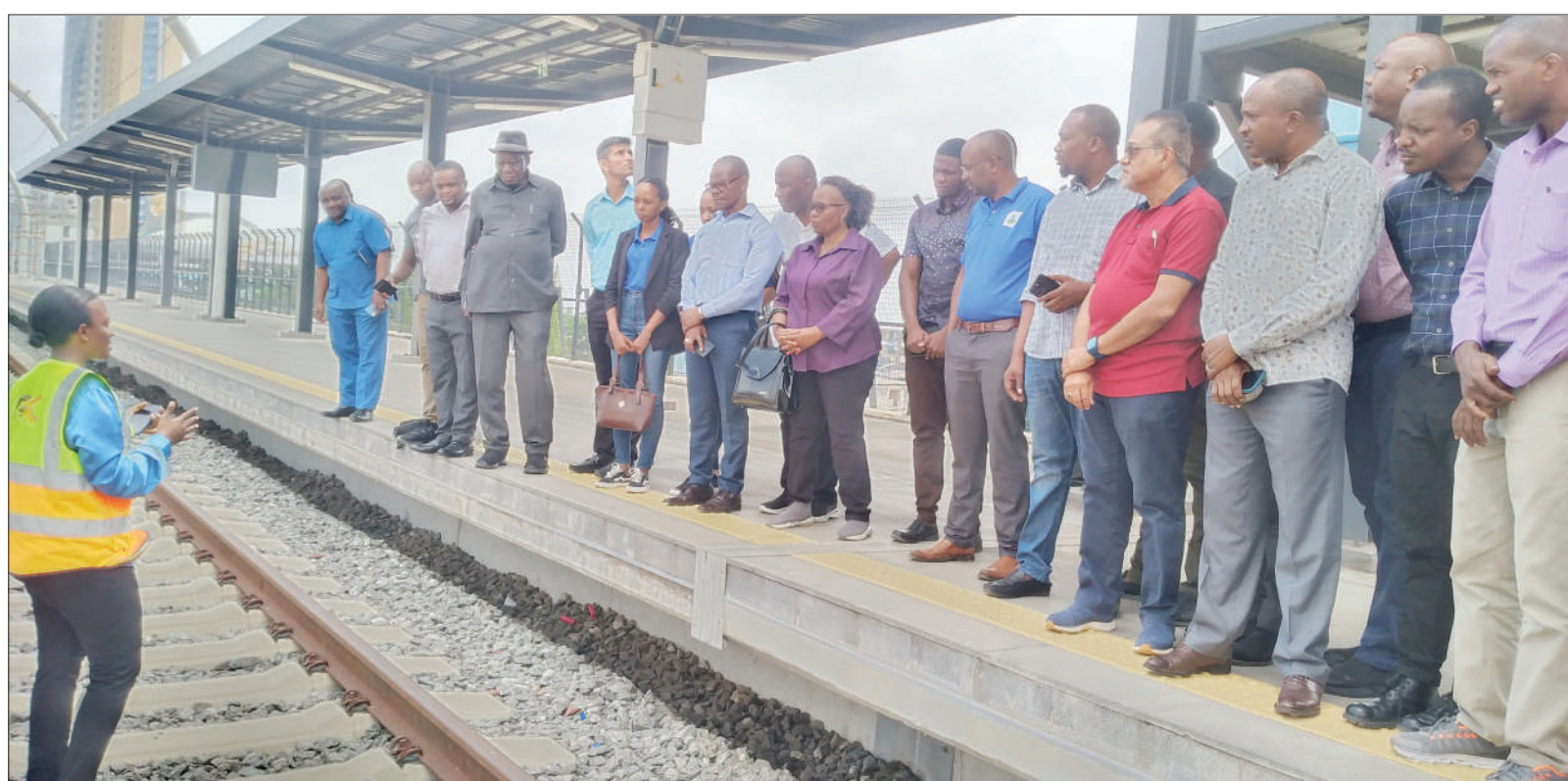
Tanzania Railway Corporation (TRC) assistant Engineer Doris Bigirwa explains to members of the Confederation of Tanzania Industries (CTI) about the progress of the construction of the Standard Gauge Railways (SGR) when they visited the project yesterday from Dar es Salaam to Kwana Dry Port. Photo: Correspondent Joseph Mwendapole
