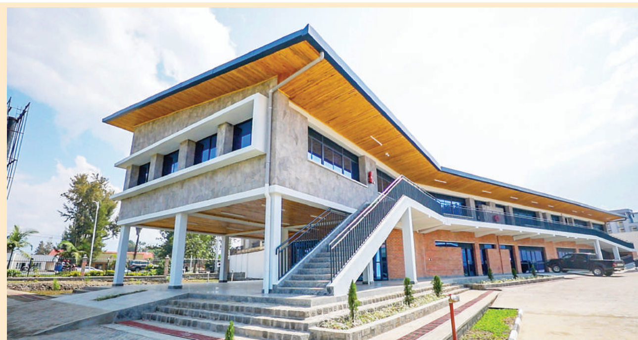
A view of Musanze's newly renovated youth centre for nurturing a dynamic and skilled young generation.
