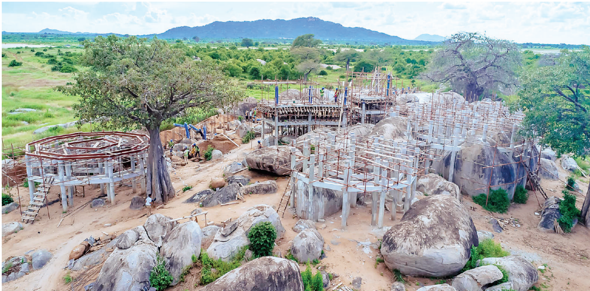
On-going construction of an information centre at the Ruaha National Park
