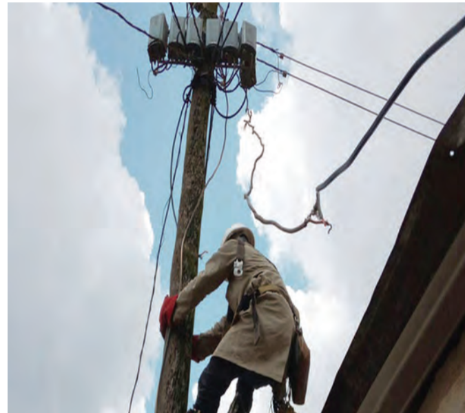
An engineer disconnects illegal electricity users.
