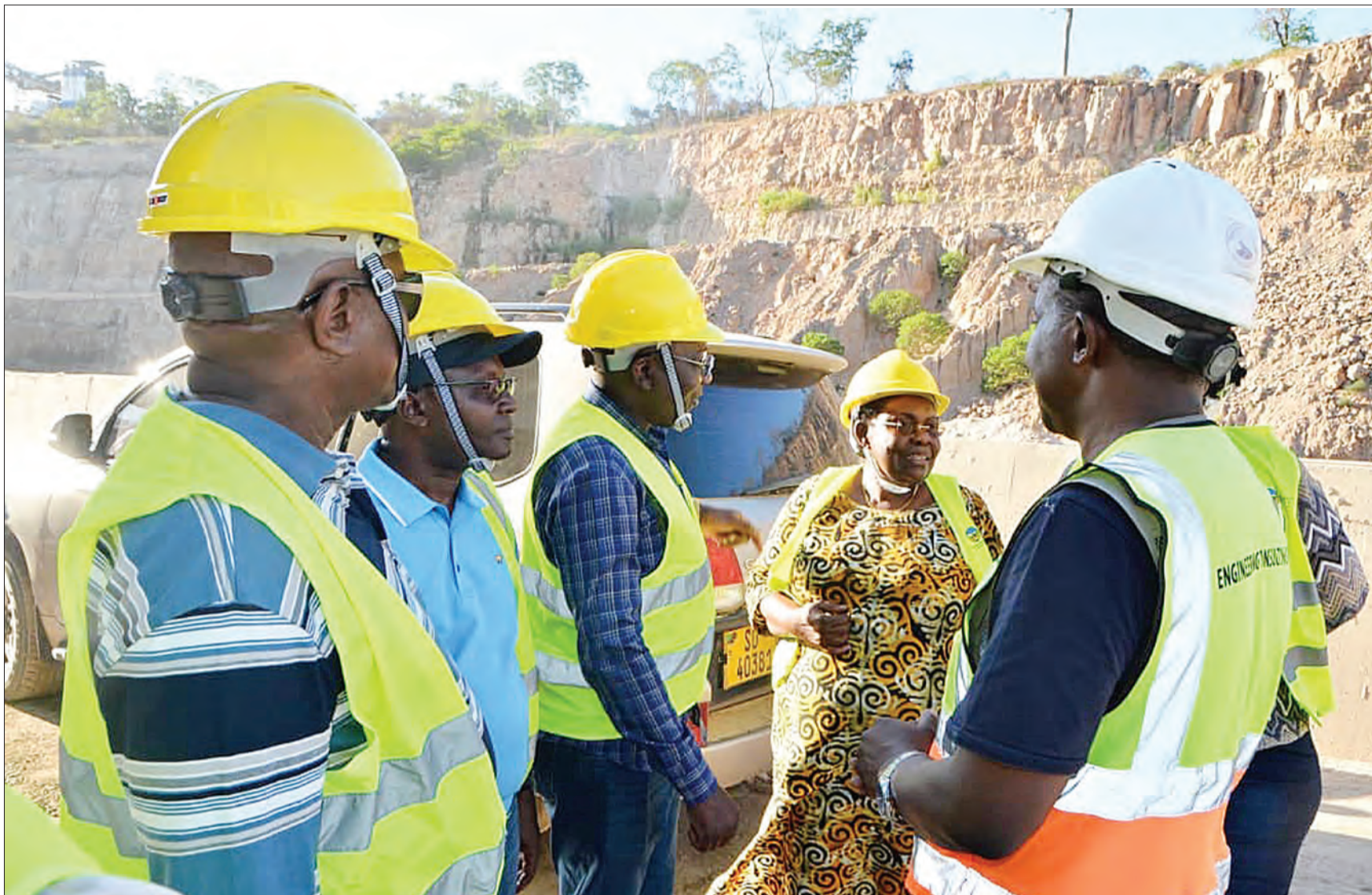
Contractors Registration Board chairperson Consolatha Ngimbwa (4th-L) makes remarks when members of the board toured the Julius Nyerere Hydropower Project in Rufiji District on Friday. Third left is CRB registrar Rhoben Nkori. Photo: Correspondent Miraji Msala
