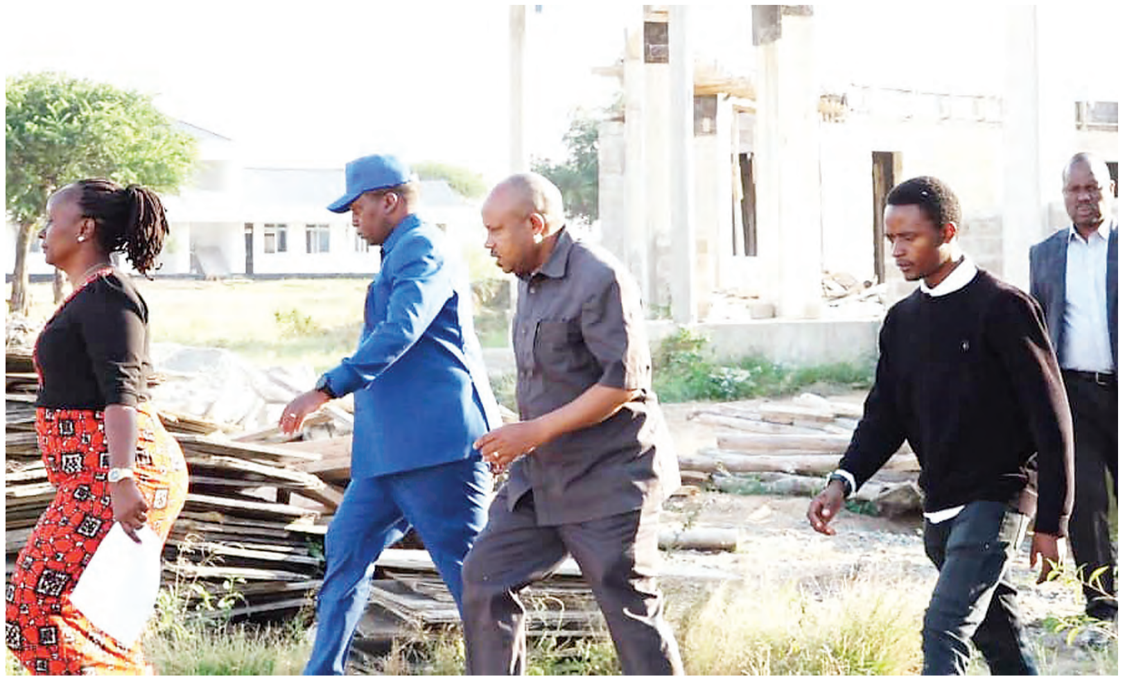
Mara regional commissioner Col Evans Mtambi (in cap) accompanied by Bunda district commissioner Dr Vincent Naano (3rd-L) when inspecting progress in the construction of a girls' secondary school at Bulamba village yesterday in preparation for the enrolment of Form Five students. Others are the school's headmistress, Nyaeri Mwisawa (L); Mara regional administrative secretary Gerald Kusaya (R) and the site construction manager, Timothy Mwanjala. Photo: Guardian Correspondent
