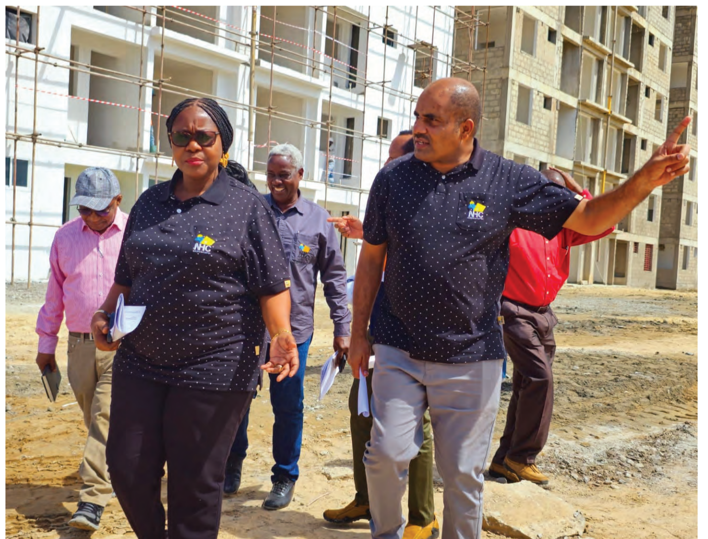
National Housing Corporation director general Hamad Abdallah takes around in Dar es Salaam on Thursday with the agency's board members, who were on an assessment tour of progress in the ongoing implementation of the Samia Housing Scheme project. Photo: Correspondent Joseph Mwendapole
