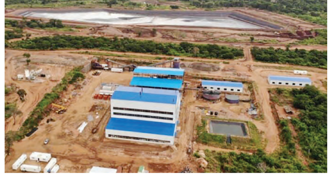
Aerial view from the south of the Lindi Jumbo processing plant with the TSF in the background
